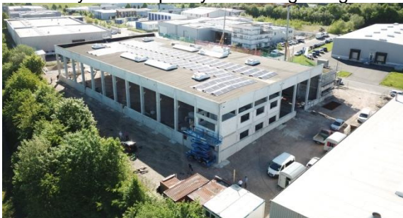
New building knife factory Germany
